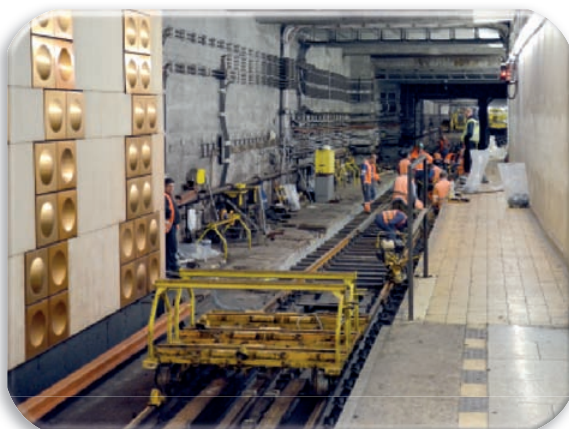
Completing work on replacing a switch at Háje station
