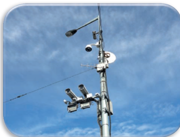
Monitoring and video detection cameras at Vypich intersection
