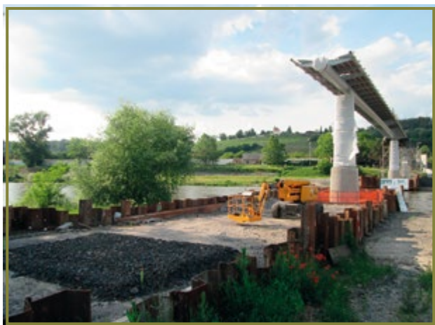
Troja footbridge after installation of the central segment
