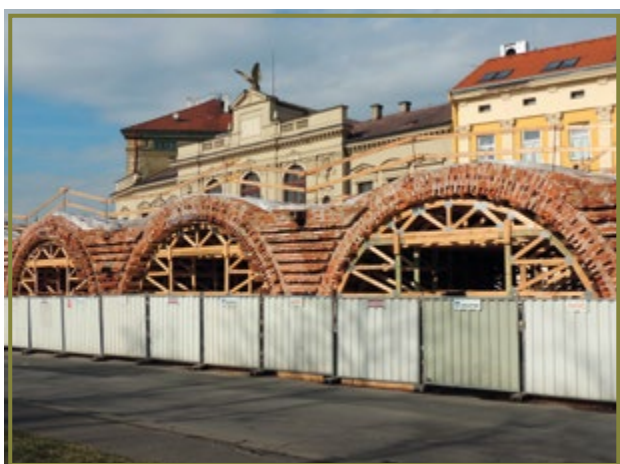
Reconstruction of Negrelli Viaduct
