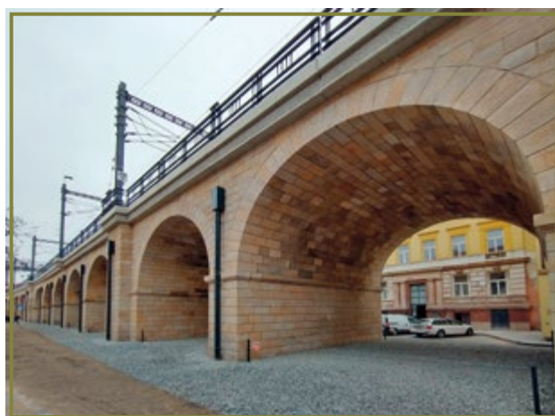
The viaduct's sandstone arches following repairs
