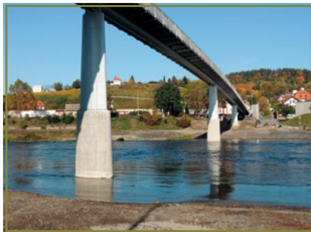
The new Troja footbridge after completion
