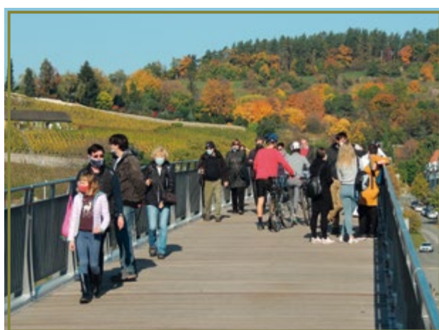
New Troja footbridge
