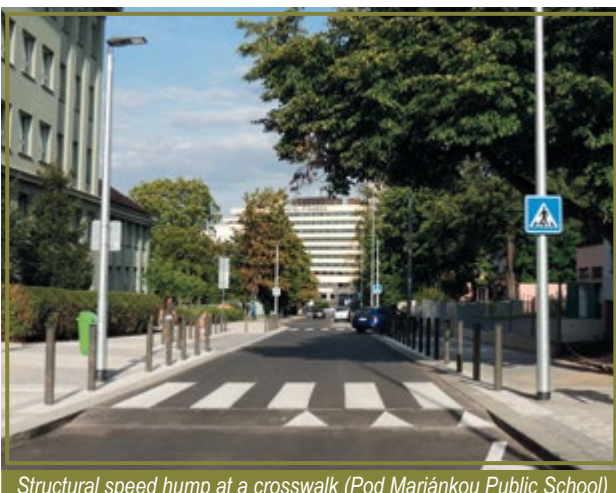
Structural speed hump at a crosswalk (Pod Marjánkou Public School)
