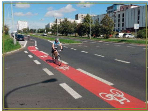
The Novodvorská bicycle lane
