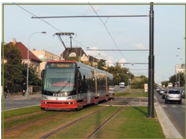
Reconstructed tram track in street V Olšínách
