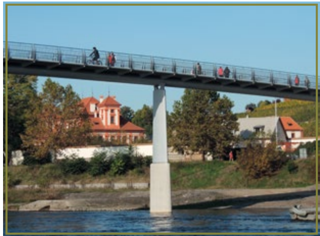
The Trojan footbridge in the 2020 budget claimed CZK 140 million
