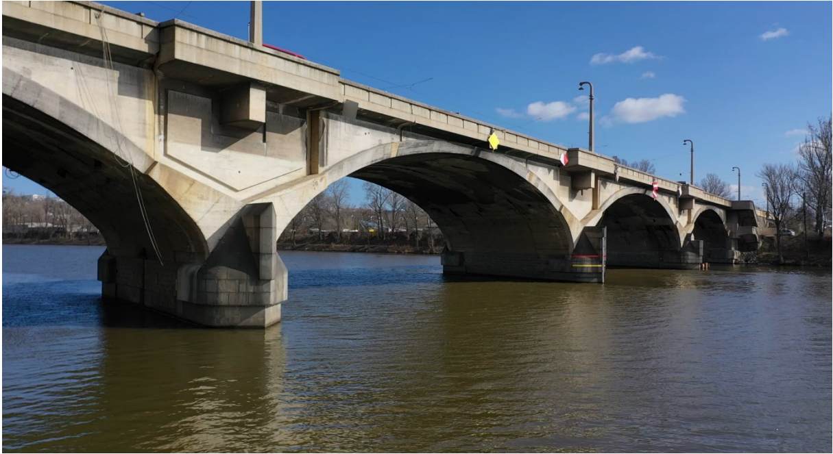
Side view of the bridge No. V009 across the Vltava
