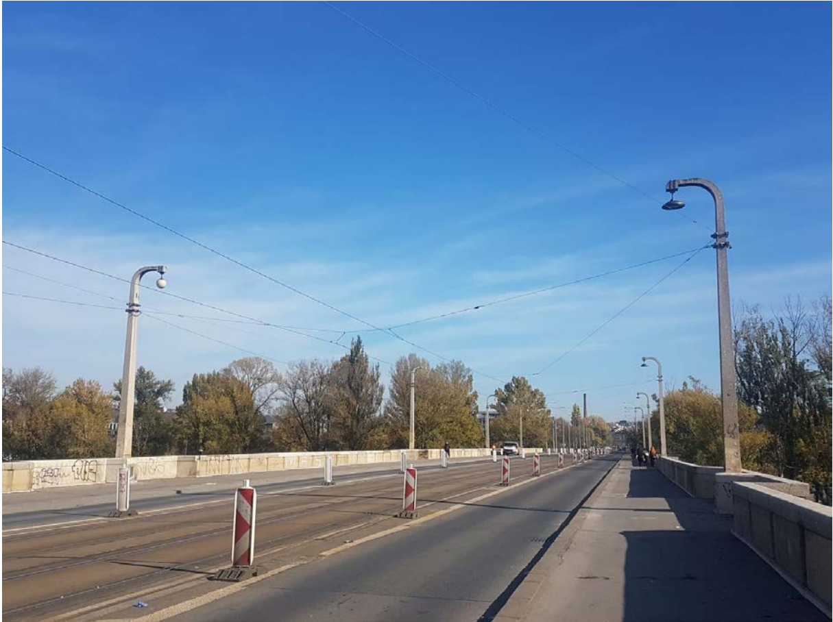
View of the bridge roadway, historical lamp posts
