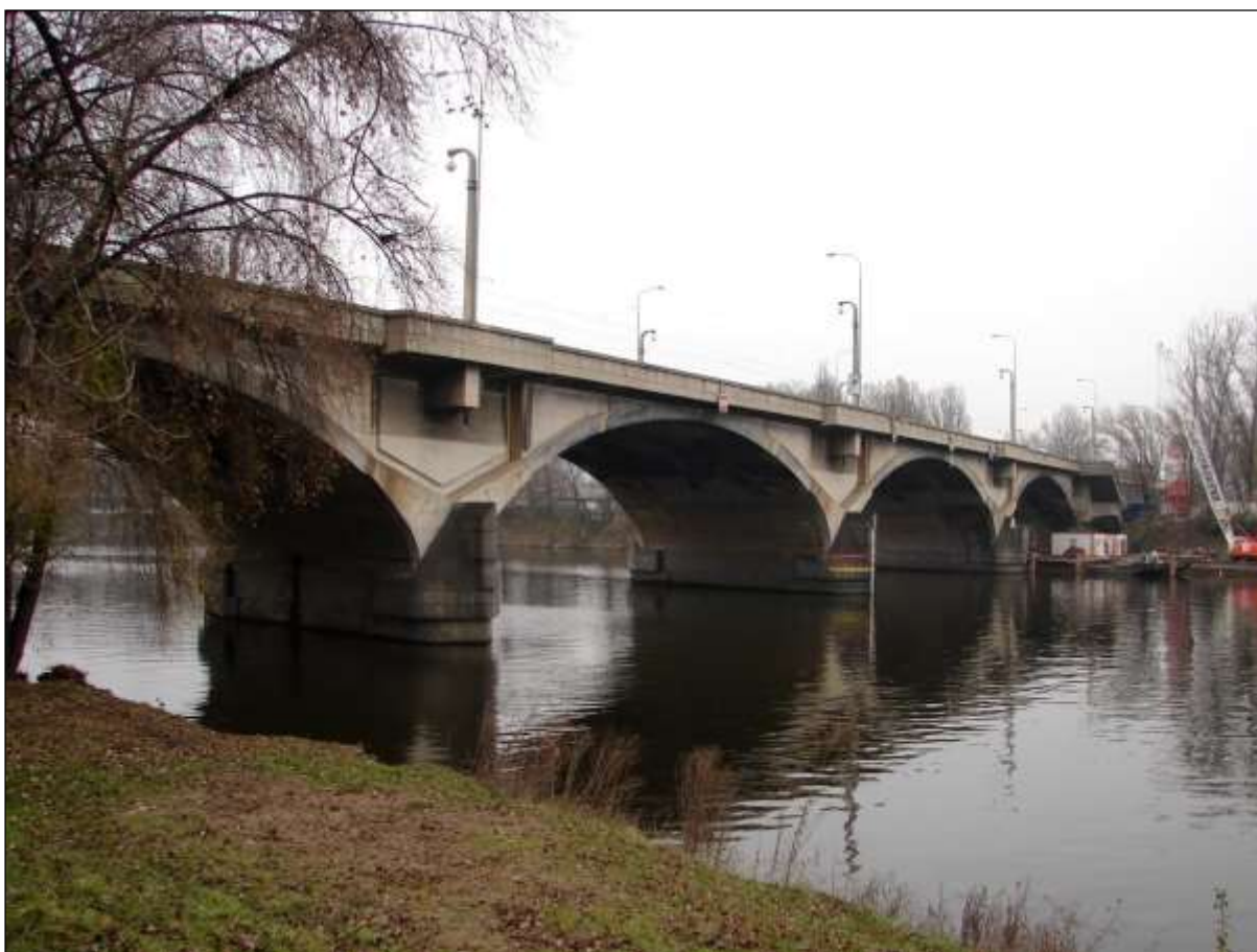
Fig. 1: View of the Libeň bridge
