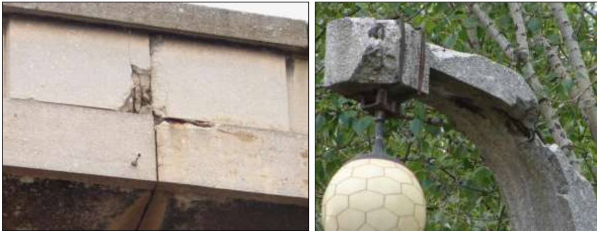
Fig. 12 and 13: Damage in the railings and cantilevers in the upper part of the vault caused primarily by dilation. Damage of the street lamp post caused by reinforcement corrosion and weather conditions
