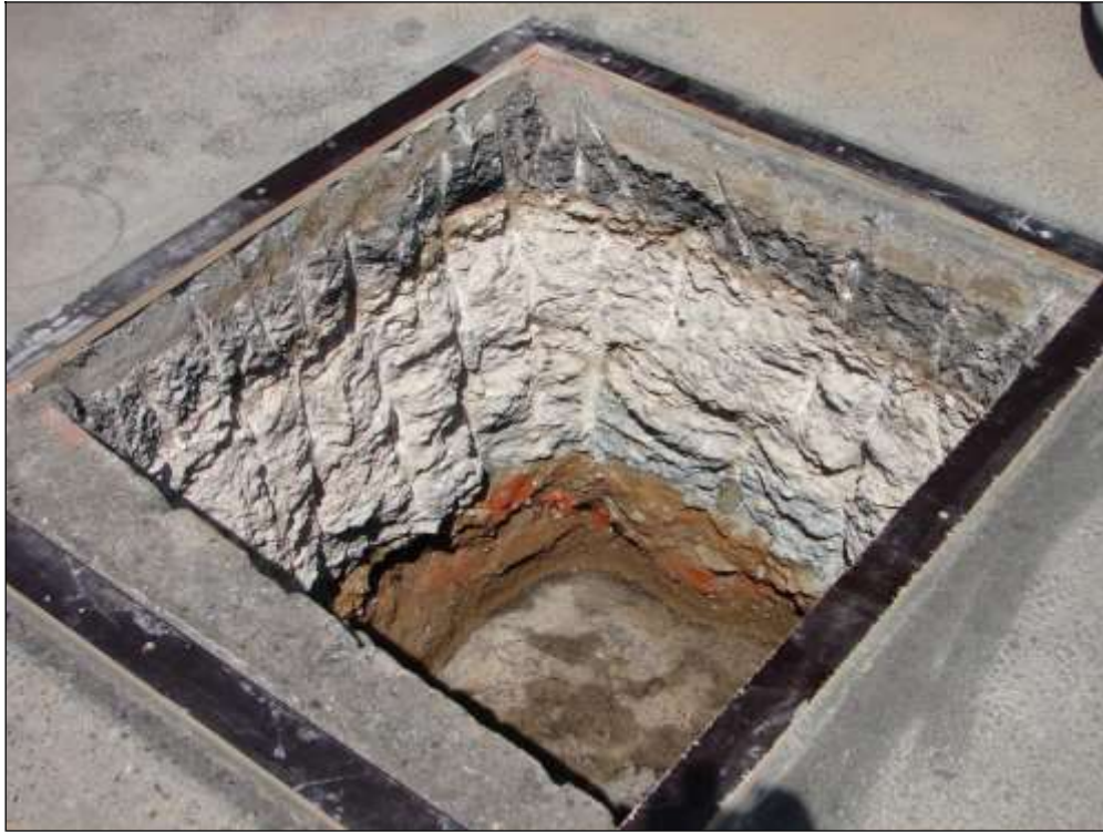
Fig 15: Concrete layers underneath the roadway of the vault part and backfill consisting of gravel sands and building debris
