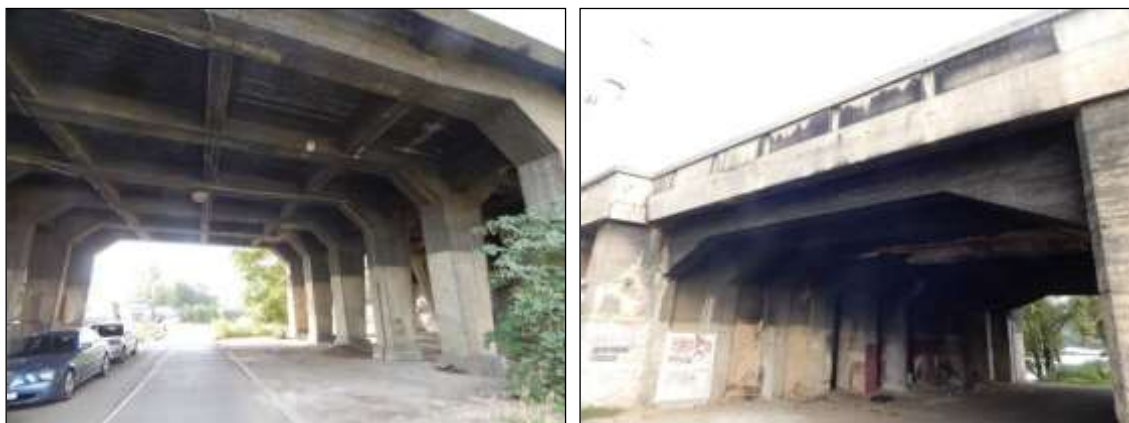
Figs. 4 and 5: Frame structures on both sides of the river (Holešovice and Libeň)
