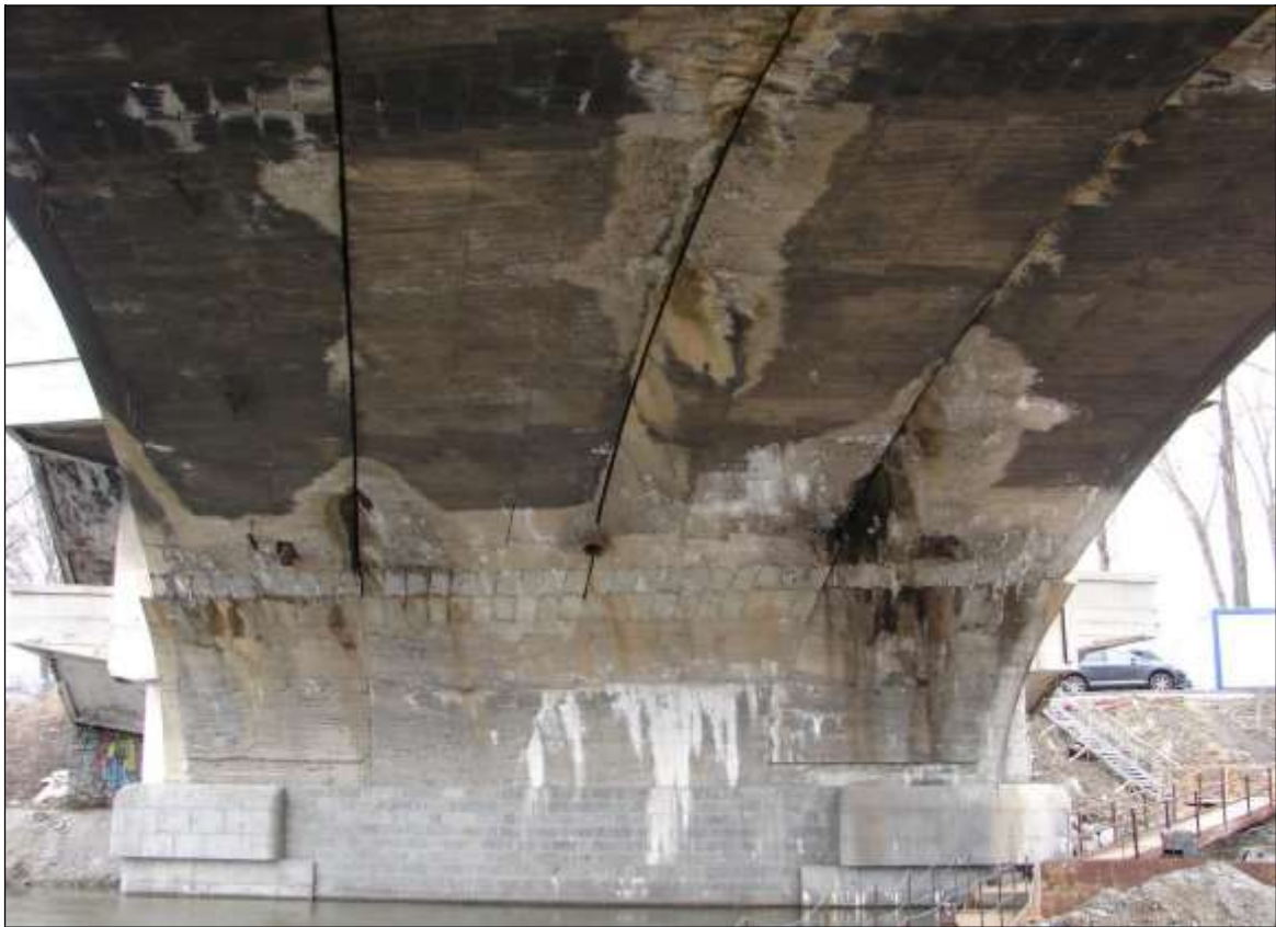
Fig. 10: Concrete degradation in the vaults and abutments caused by water leakages in conjunction with frost
