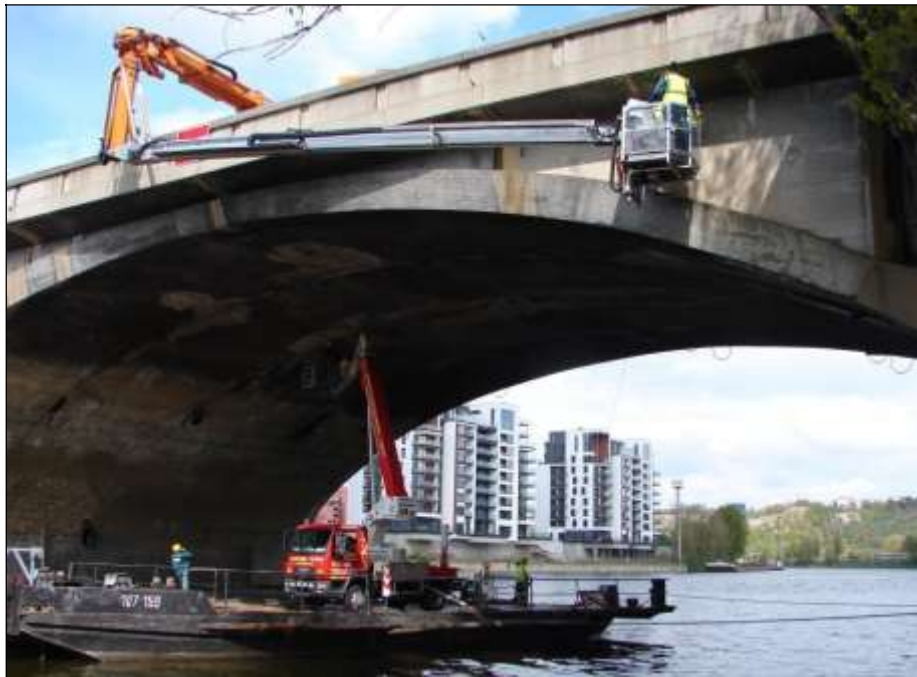
Fig. 6: Diagnostic inspections of the bridge structures
