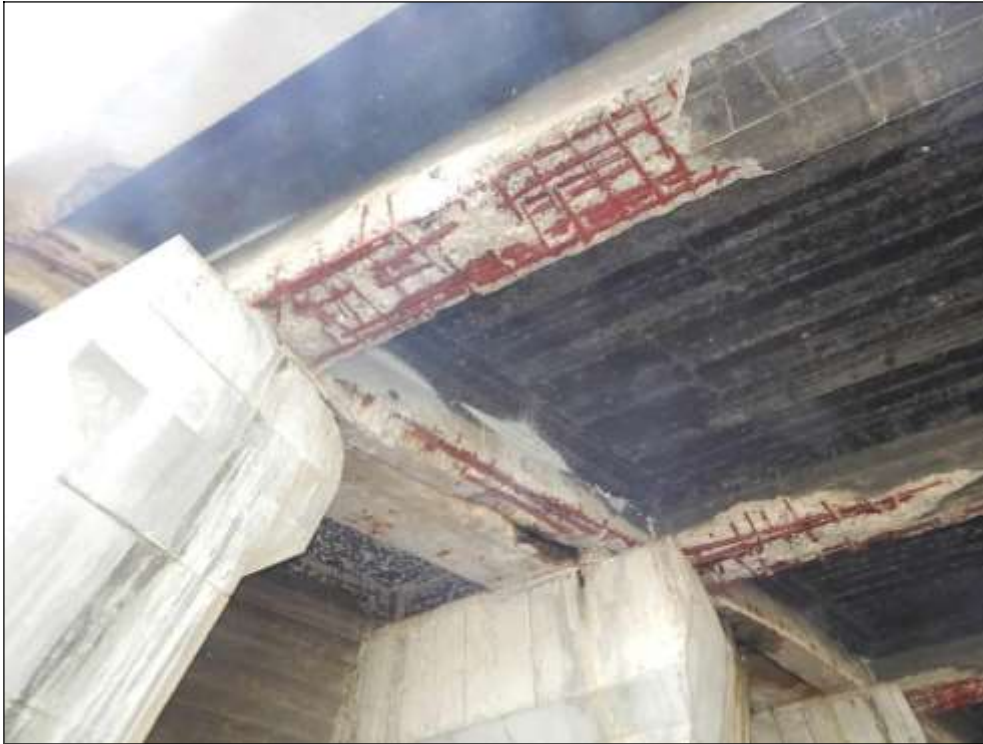
Fig. 17: Frame structure; Holešovice frame part, part I-VI in the joint area; weakened reinforcement and deep degradation of concrete - emergency condition
