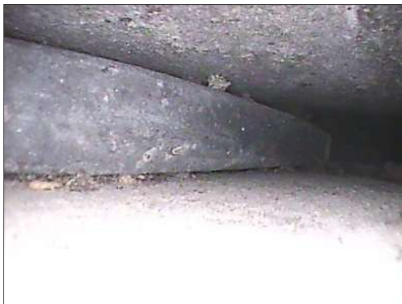
Fig. 11: Plumb slabs in the vault joints without any apparent damage
