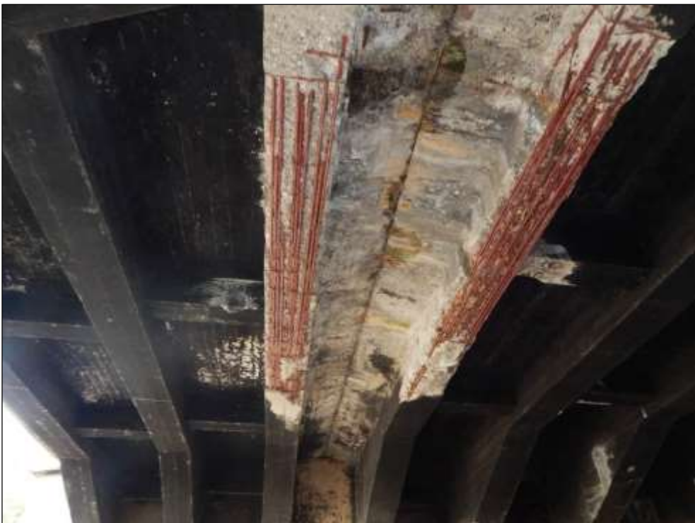
Fig. 18: Frame structure; Libeň frame part, part C in the area along the expansion joint; weakened reinforcement and deep degradation of concrete - emergency condition
