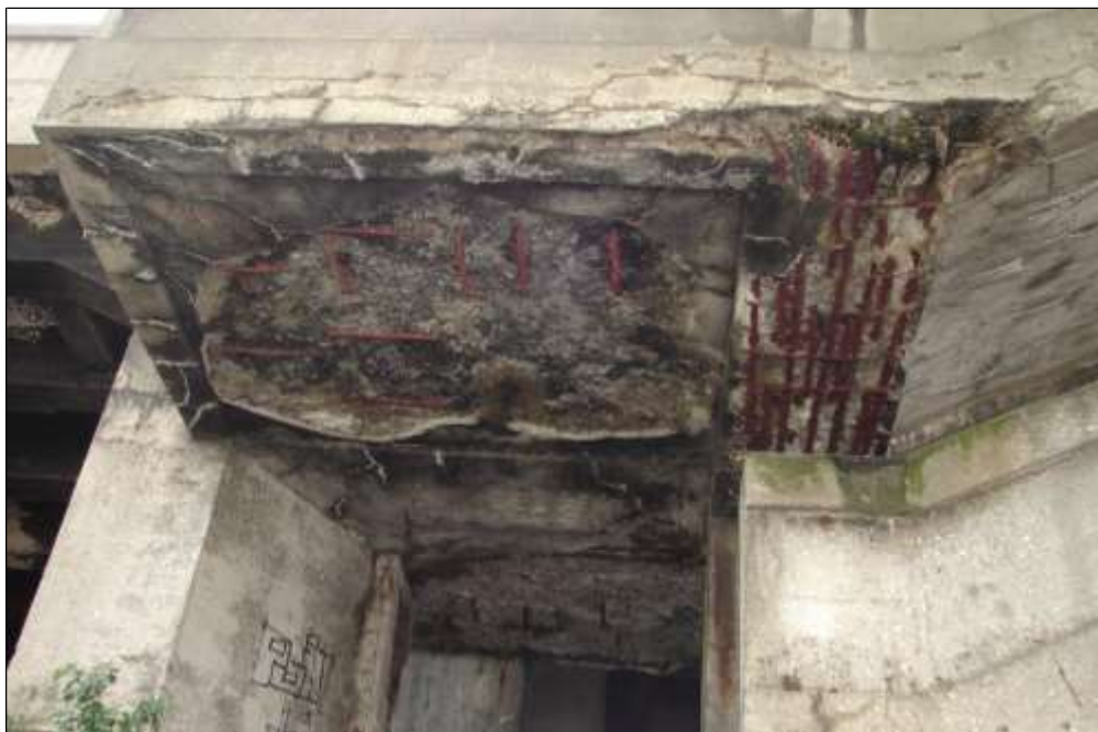
Fig. 16: Staircases; weakened reinforcement and deep degradation of concrete - emergency condition
